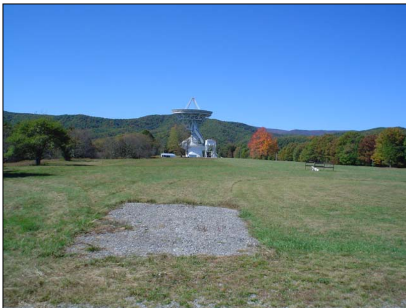
Figure 7: View Towards the North
